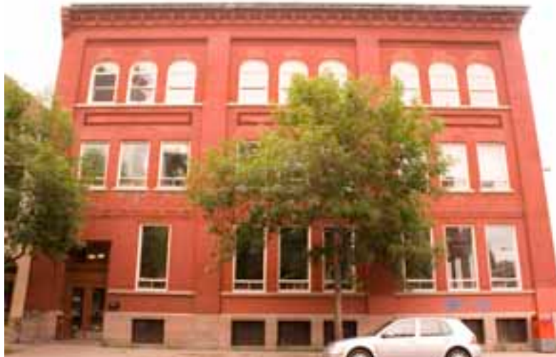
This building is a 3-storey brick loft with finely-detailed facades. In good condition, it serves a national food-catering business.
