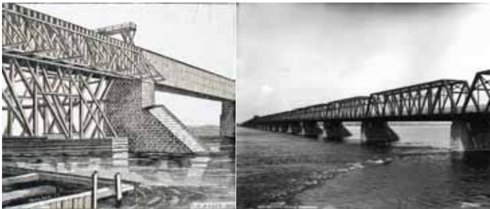
Figure 2.22: Composed of a metal tube supported by limestone piers, Victoria Bridge would be described as the “eighth wonder of the world” in 1873. McCord Museum.
